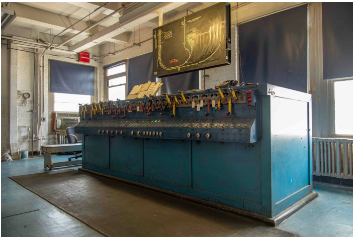
The 55-lever US&S Model 14 machine in Tower B.
