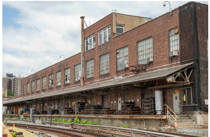
Tower B, at the extreme north end of the yard, is what occupies the third floor of this building, which houses the 215th Street Signal Shop.
