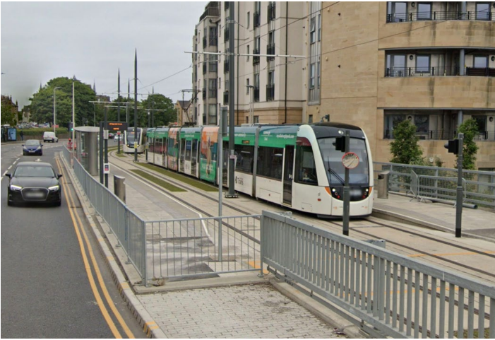
The new terminal station at Newhaven in June. Google street view
