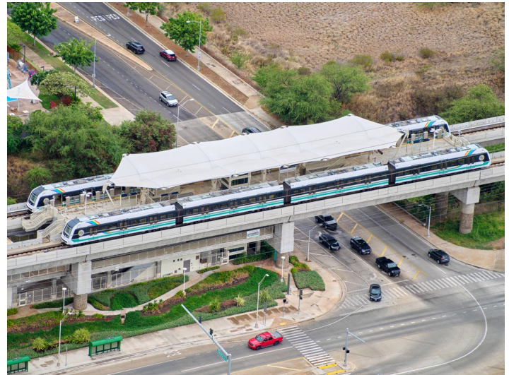
Aerial view of the Kualakai-East Kapolei Station late last summer, on September 15, 2022. HART photo
