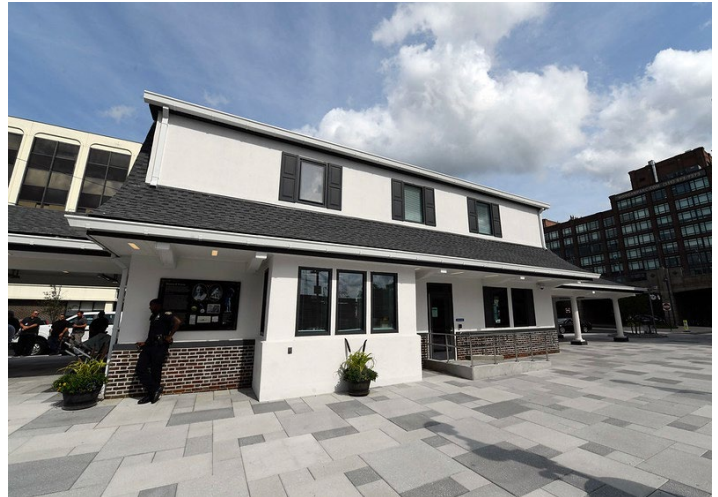
Mineola station building on September 22, 2023. Marc A. Hermann/MTA photo
