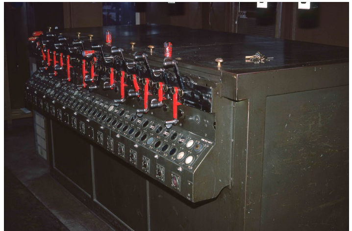
In Valley Tower on January 8, 1978, the original US&S 35-lever Model 14 interlocking machine was still in everyday use. Jeff Erlitz photo
