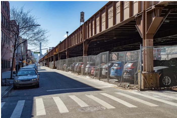
View looking south from the east side of Park Avenue at 122nd Street at the existing structure. Trent Reeves photo
