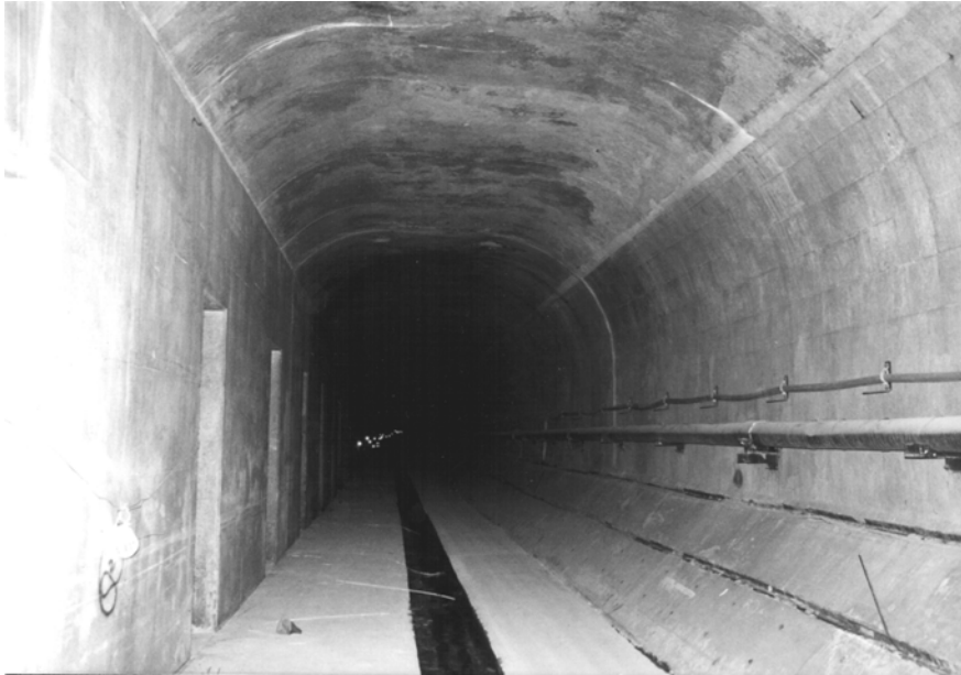
63 rd Street Tunnel, LIRR Level — Westbound trackway looking west in the immersed tube section under the East Channel of the East River
