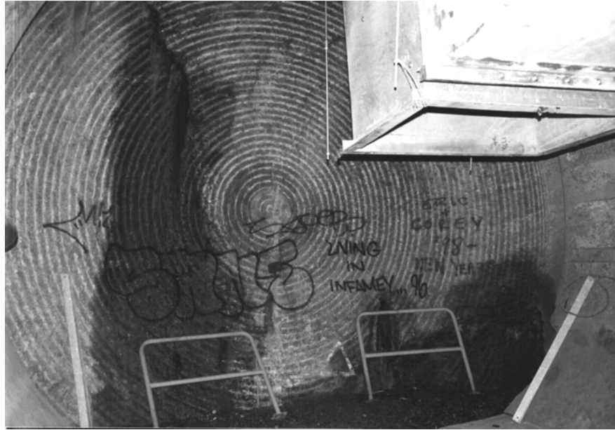
63 rd Street Tunnel, LIRR Level — Bulkhead of the westbound trackway 150 feet below Second Avenue
