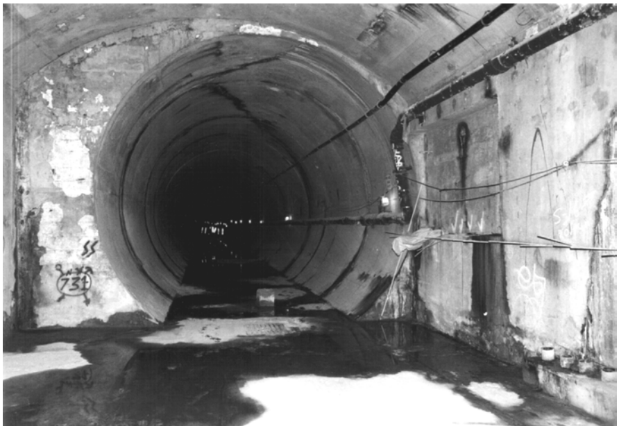
63 rd Street Tunnel, LIRR Level — Westbound trackway looking west at the start of the bored section, York Avenue in Manhattan
