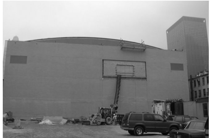
The Ninth Avenue side of the building. Note the temporary opening on the third level for delivery of equipment.
