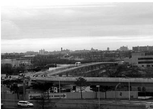
Test train on structure.
