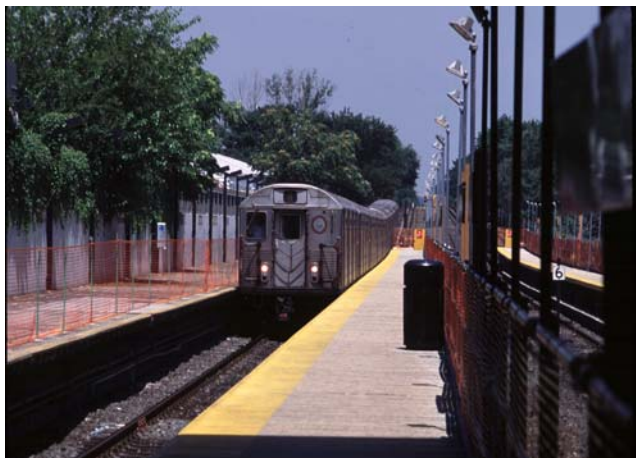
The temporary southbound platform at Howard Beach, built to facilitate Airtrain construction, is evident in this July 8, 2002 shot of R-38 4100.
