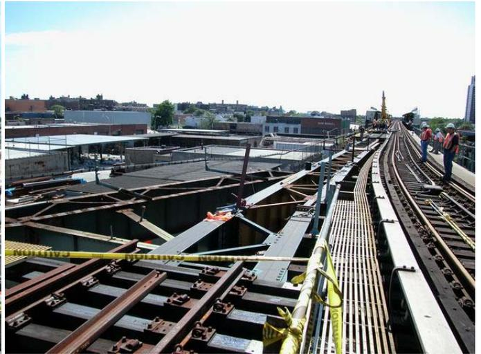
New steelwork for Track Q2 meets the existing portion of Track Q2 north of Sutter Avenue.
