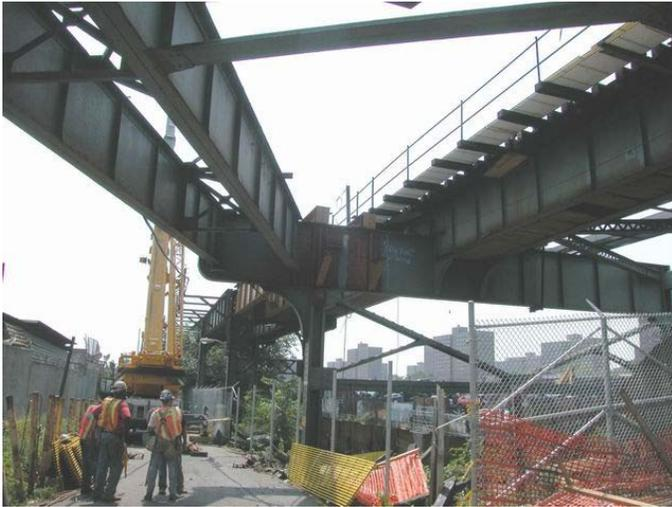
Interestingly, steel shims were installed on top of the northernmost girders of the original structure before the changeover point (see image below) to provide a smooth gradient from the original structure to the new structure. As you can see from one of the images below, several pieces of original Fulton Street EI steelwork had already been removed from above former Track P2. This work had been done sometime in the past two years.
