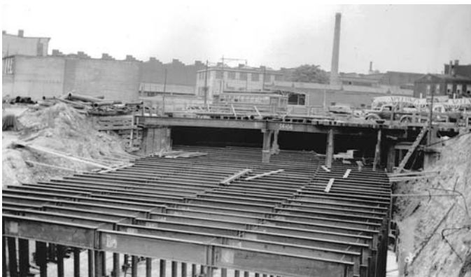
This May, 1940 photograph shows subway construction at Jamaica Avenue and Williams Place in Brooklyn. Jamaica Avenue car 1176 crosses above.
