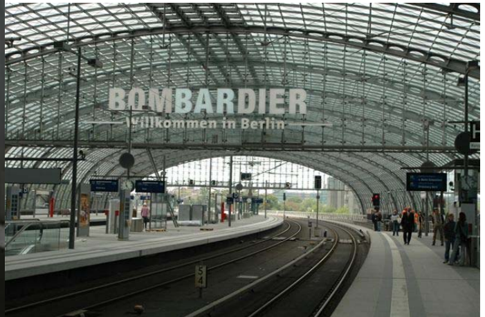
View of the train shed looking west. The S-Bahn platform is to the right with its third rail-equipped tracks. The train shed does not completely cover the long distance and regional train platforms, apparently as a cost-saving measure. It does, however, cover the shorter S-Bahn platform. I believe S-Bahn trains are currently limited to eight cars.
