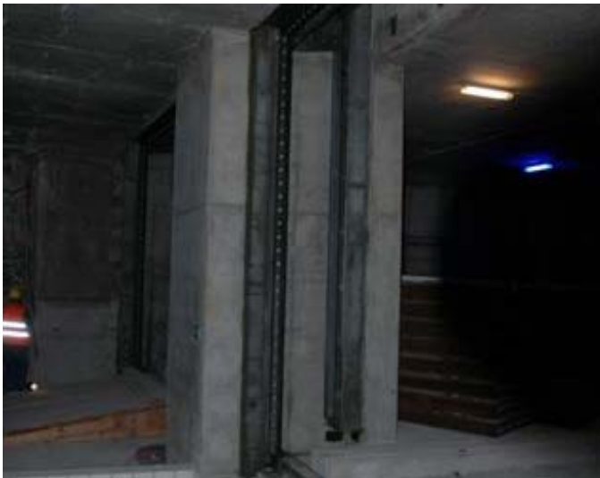
The line passes under the Spree River, and this is one of the two sets of floodgates that could be lowered should there be a tunnel breach.
