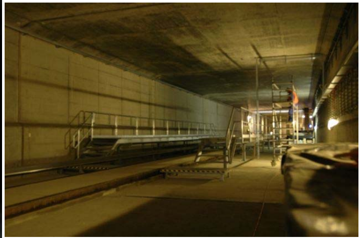
Temporary inspection area north of Hauptbahnhof station. The single track is temporarily centered in the subway structure.
