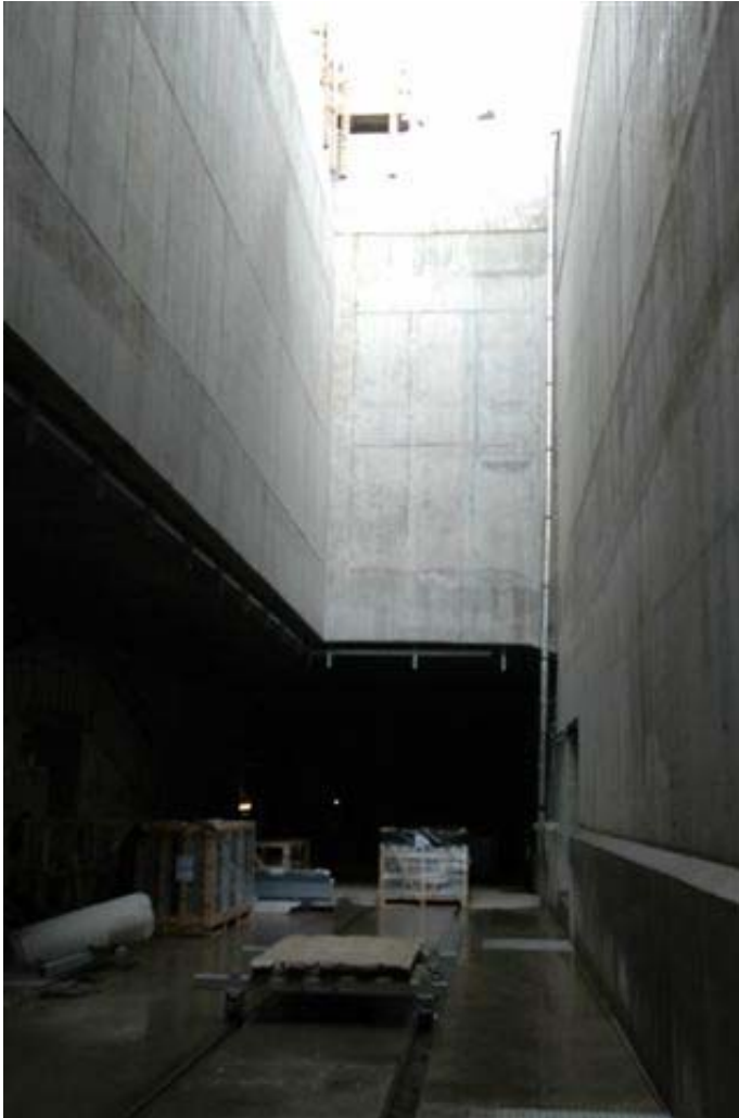
Access shaft for the delivery of all equipment, including the subway cars. This is just long enough for one subway car without its couplers. All of the material for the construction of the second track has already been delivered and stacked up on the right of way of the future track.
