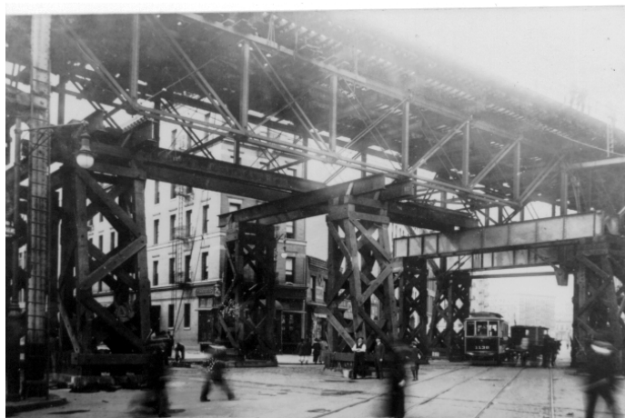
Eighth and St. Nicholas Avenues at W. 122 nd Street, October 19, 1915. The structure is being reinforced for addition of a center express track. A 110 th Street battery car is in the background.
