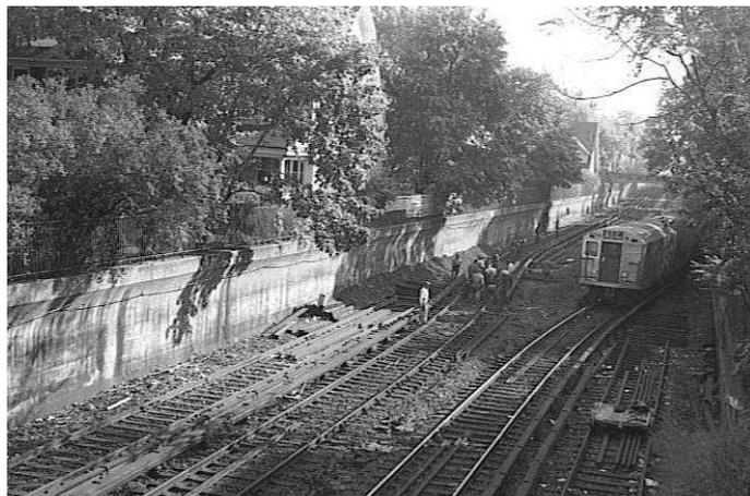
Temporary tracks during construction of platform extensions at Newkirk Avenue, looking south from the Foster Avenue Bridge on October 14, 1964. Note the train of brand-new R-32 cars.
