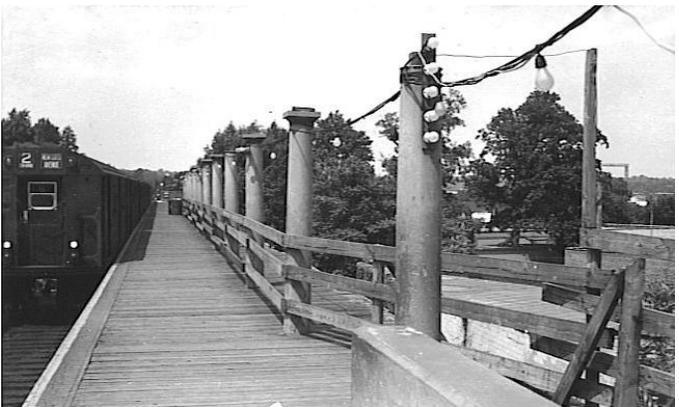
**Dyre Avenue station on June 20, 1959, showing temporary repairs made after strong winds blew off the platform roof.**
