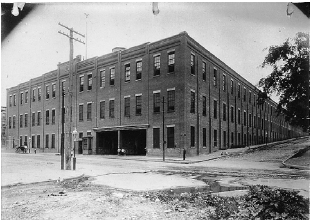
58 th Street Depot, Second Avenue and 59 th Street.
