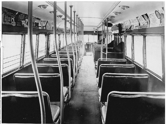
PCC 1001, showing stanchions near each seat on the left side.
