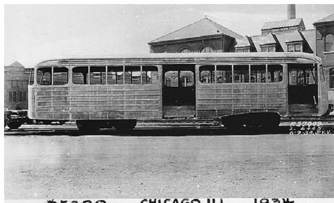
#5300 CHICAGO, ILL. 1934 Frame of PCC Model B (car 5300) in Chicago in 1934. Bernard Linder collection
