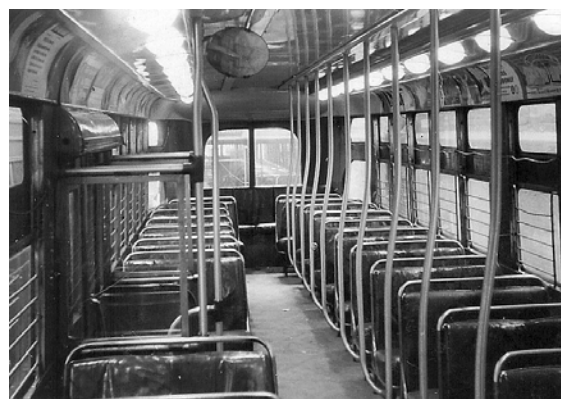
Interior of car 1000, taken in Ninth Avenue Depot on February 18, 1955. Bernard Linder photograph
