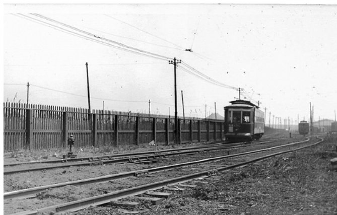
Car 4702, seen looking south from Skidmore Avenue, on March 27, 1941.
