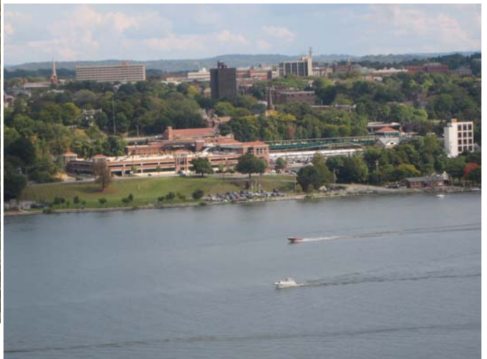
Poughkeepsie station from west side of Hudson River.
