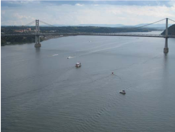
Looking south at the Mid-Hudson Bridge.
