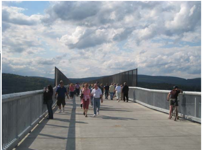
Bridge walkway, looking west.
