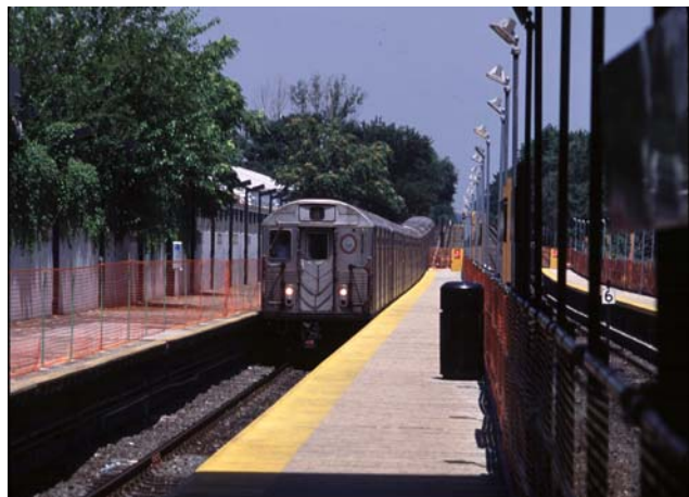
The temporary southbound platform at Howard Beach, built to facilitate Airtrain construction, is evident in this July 8, 2002 shot of R-38 4100.
