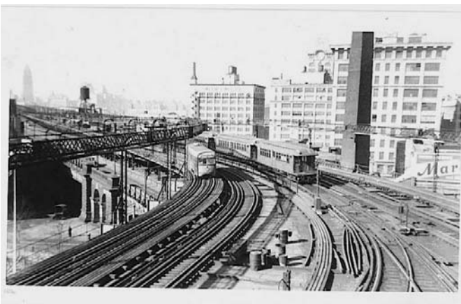
Looking west from Sands Street station, with trolley cars on the outer tracks. Bernard Linder collection
