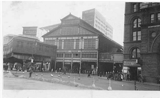
Park Row looking south, after exit platforms were removed in the mid-1930s.
