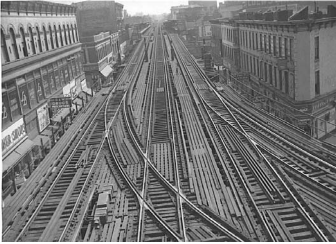
Broadway from Lexington Avenue Tower, looking east.
