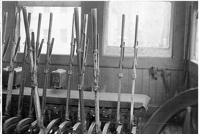
**Manual interlocking machine in South Ferry Tower.**
