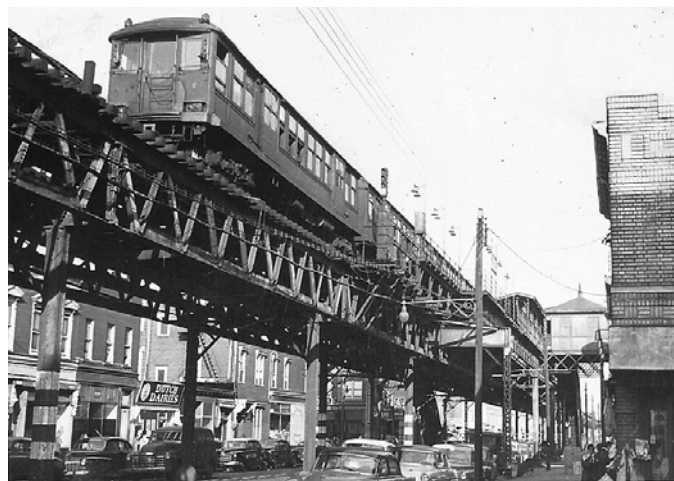
Southbound train approaching Montauk Avenue station, Fulton Street El, March 5, 1956.
