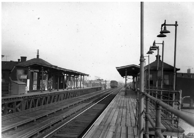
Van Siclen Avenue station, Fulton Street El, looking east, March 1, 1956.
