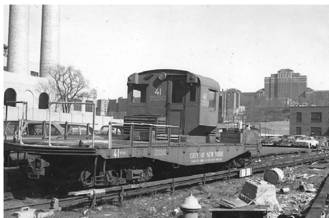
Motor flat 41, 207 th Street Yard, March 22, 1963. Bernard Linder photograph
