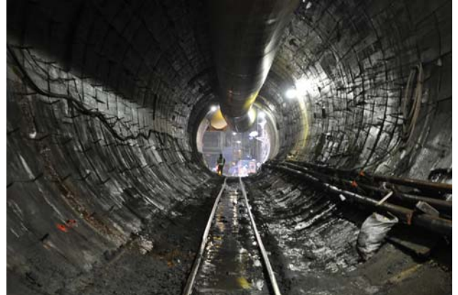
View north from inside the northbound S2 tunnel, south of E. 93 rd Street.
