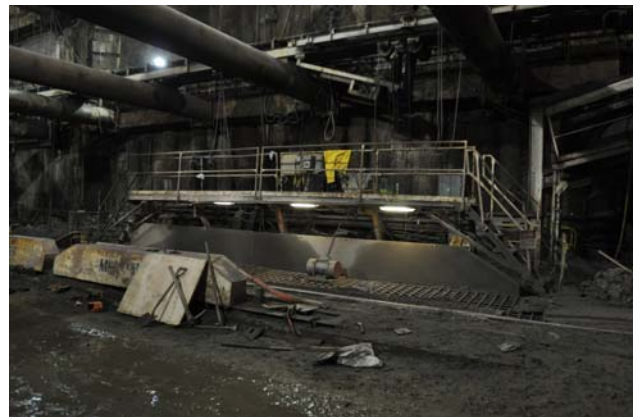
This is the muck conveyor system at the bottom of the launch box. Hopper cars filled with muck from the tunnel boring and mining operations are unloaded here and this system brings the muck up to the surface where it is loaded onto trucks for the trip to the disposal site.
