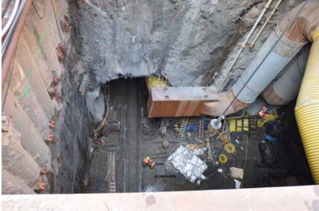
Looking down into the launch box from street level at Second Avenue and E. 93 rd Street. The tunnel for northbound track S2 is just to the left of the center.
