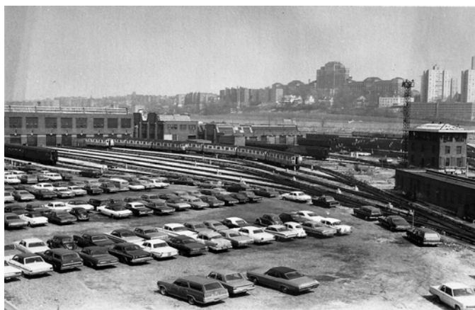
207 th Street Yard, April 4, 1969.
