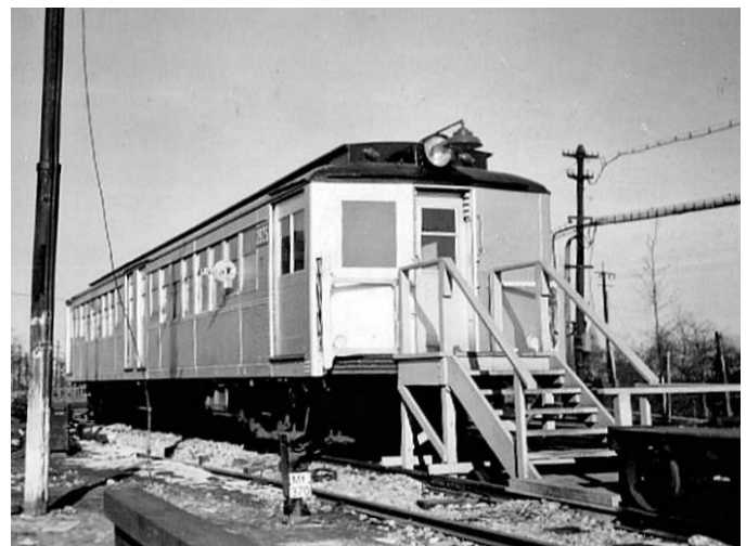
NYCT car 2925T (ex-SIR 504) serving as an office in Fresh Pond Yard, March 3, 1957. Bernard Linder photograph
