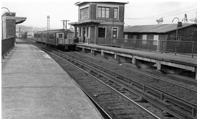
Clifton station, looking north, October, 1968. Larry Linder photograph
