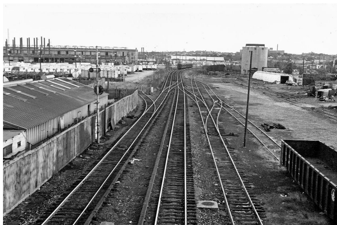
Looking south from Tompkinsville station, October, 1968. Larry Linder photograph
