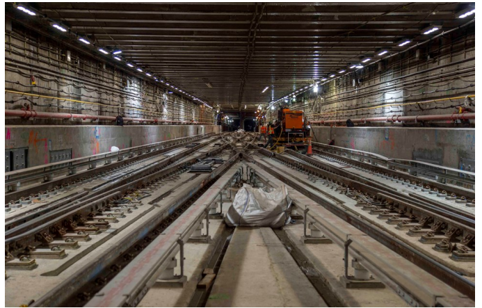
Looking east at GCT-6 Interlocking under 63rd Street. I believe this is directly under the IND 63rd Street Line's FDR Drive Interlocking. At the far end of the crossovers is the FDR Drive ventilation shaft and emergency exit.
