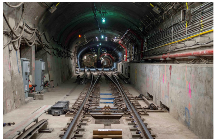
Looking south at switch 542 in GCT-5 Interlocking. Track EB4 from the upper level is at the left and Track EB2 from the lower level is on the right. You can see the grade changes to the upper and lower levels in the distance.
