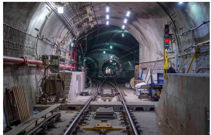
View south on Track EB4 at GCT-3 Interlocking. This is the east-bound track to Queens. You can see the westbound track from Queens on the right in the cavern up ahead at the double crossover. All the signals at five of the six "GCT" interlockings are already energized. The signal equipment was supplied by Union Switch and Signal (Hitachi STS these days) and are Style M-3 switch machines and Transit signal heads.
