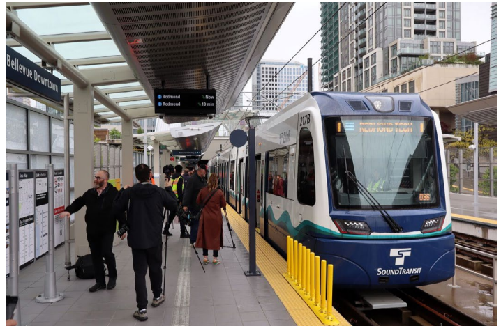
Downtown Bellevue Station on April 26, the day before the official opening. Doug Trumm/The Urbanist photo
