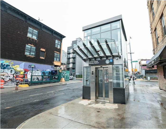
View south towards the new street-to-mezzanine elevator just off the northwest corner of Lorimer Street and Metropolitan Avenue on April 1. Marc A. Hermann/MTA photo
