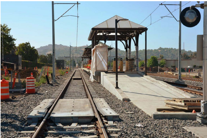
View southeast of Glendora Station from S. Vermont Avenue.
