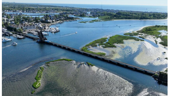
Aerial view of the Brielle Drawbridge. Hardesty & Hanover photo
