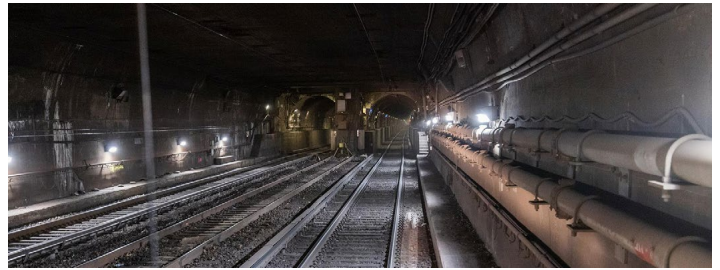
Looking east from just outside Penn Station towards, left to right, Lines 2 and 1 of the East River tunnels. Amtrak photo
