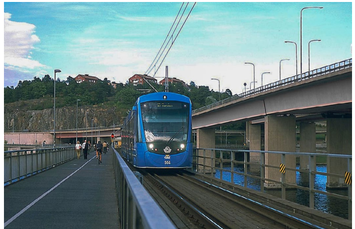
The Old Lidingö Bridge over the Lilla Vartan was converted to this bi-directional single-track configuration during the tram line's renovation between 1983 and 1985. Inbound car 551 is crawling across the 92-year old structure. All motor traffic uses the taller bridge at right.
