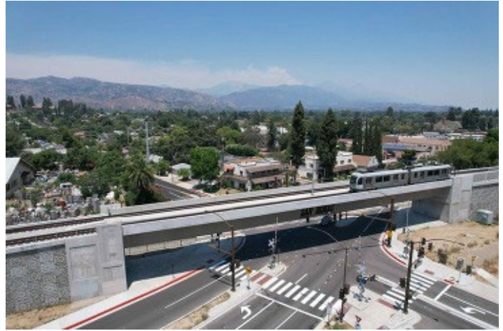
Powered light rail vehicle moving across the Bonita Avenue/Cataract Avenue light rail bridge in San Dimas.
