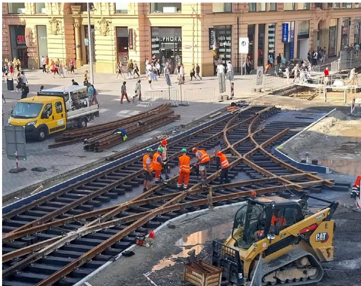
The new tram junction under construction at Wenceslas Square and Vodičková and Jindřišská Streets on August 4. This is the north end of the new tram trackage in the square and the view is looking north. Dopravářek (Transporter) photo
