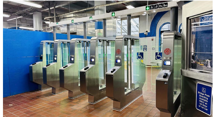
The new fare gates at the 69th Street Transit Center. SEPTA photo
