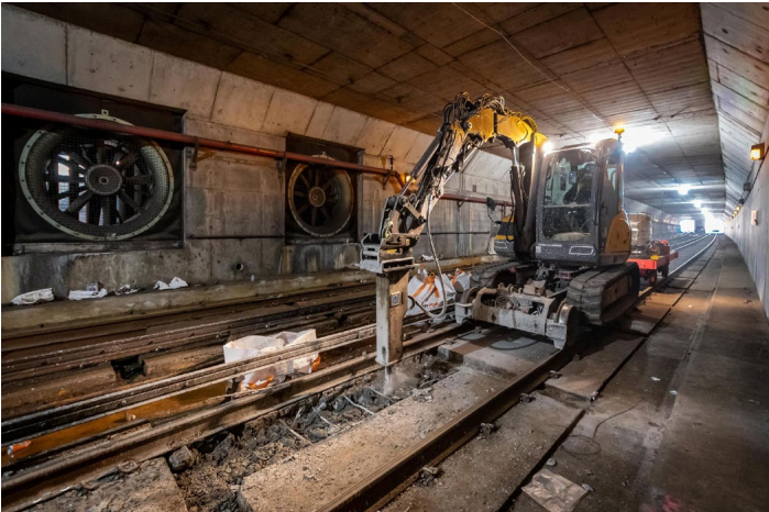
View of the track work taking place north of Massachusetts Avenue Station on the Orange Line on October 11. MBTA photo
