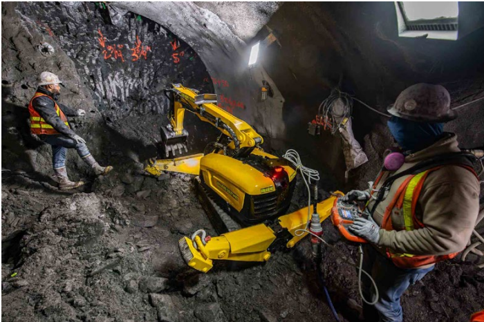
A view of the tunneling work that was required for the new passageway, taken on April 26, 2024. Trent Reeves/MTA photo
