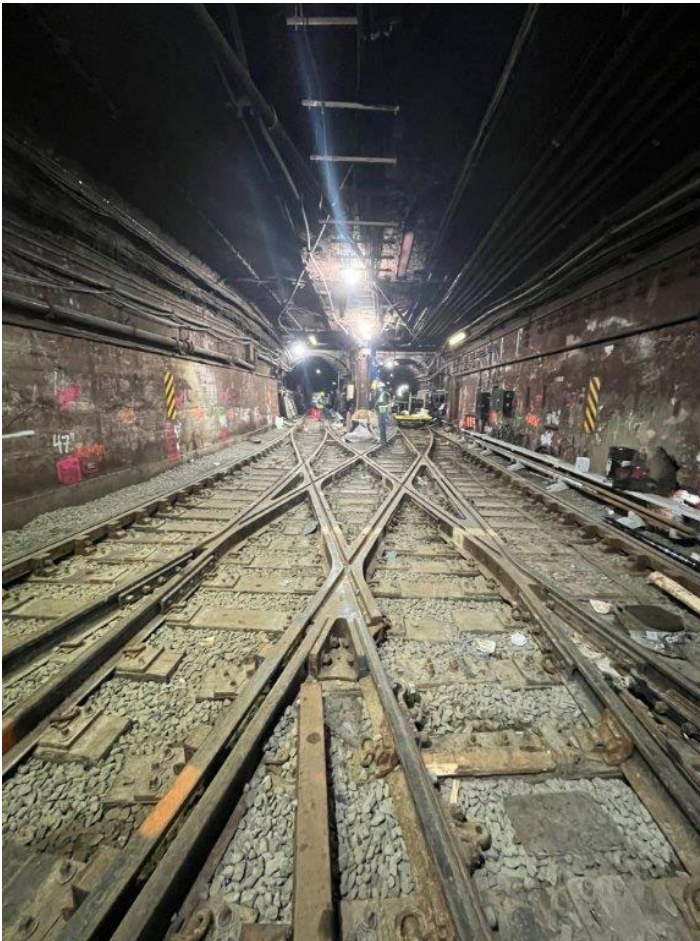
Two views of the recently completed work at Hoboken. (Above) Looking towards the station from the interlocking, where all of the track was replaced. (Below) A view of the station area, with new platform topping, staircases, painting, and lighting. PATH photos
