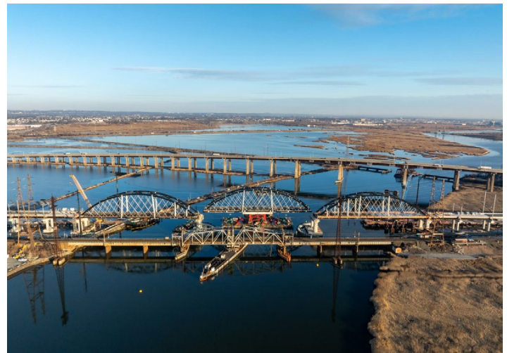
Aerial view of the Portal North Bridge with the third arch about to be placed into its final position. HNTB photo
