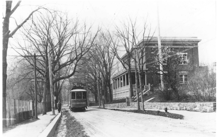
(Above) Glen Cove RR operating on the line between the Glen Cove LIRR depot and the center of Glen Cove. Note the single-track operation, pantograph for the 2.2kV AC system and the unpaved street. (Below) Glen Cove RR cars No. 402(?) and No. 404 were single- and double-truck Birney cars respectively. Location is the Sea Cliff LIRR station terminal. Both cars are equipped with pantographs for the 2.2kV AC system. Collection of the Electric Railroaders' Association, photographer and date unknown.
