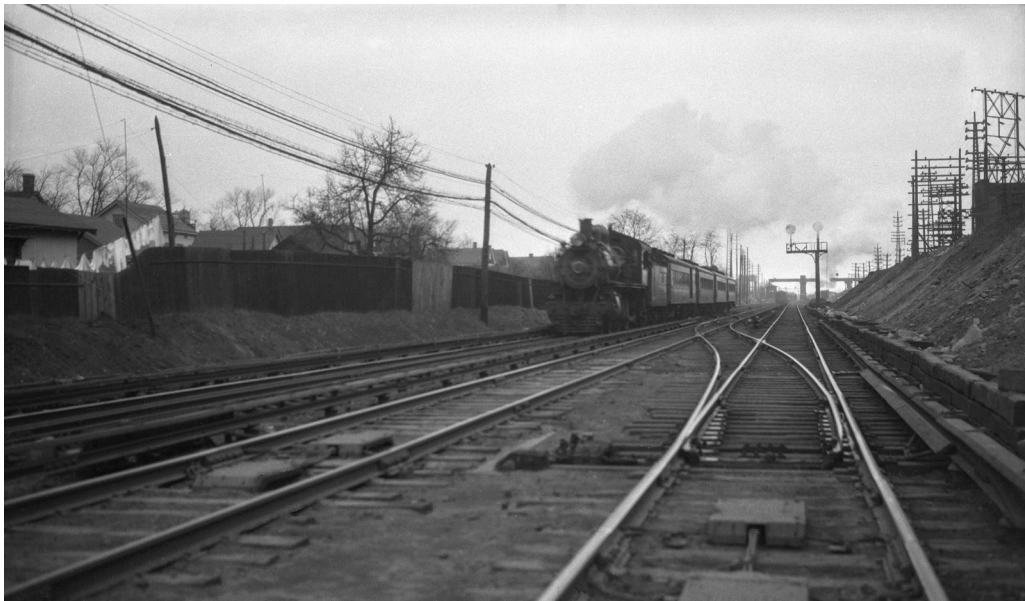
In the view above, Class G5s No. 27 (PRR-Juniata, 1/1925, s/n 3976) is leading an eastbound train on Track 3 at 159th Street. The track immediately to the right of the train stub-ended at the high-level platform of Union Hall Street Station. The temporary J1 Block Station is barely visible on the right, through the signal bridge. Below, class D16sb No. 223 (PRR-Juniata, 2/1906, s/n 1444) leads a westbound train through the switches of J2 Block station, at 170th Street. The overpass in the distance is at Hillside Station.
