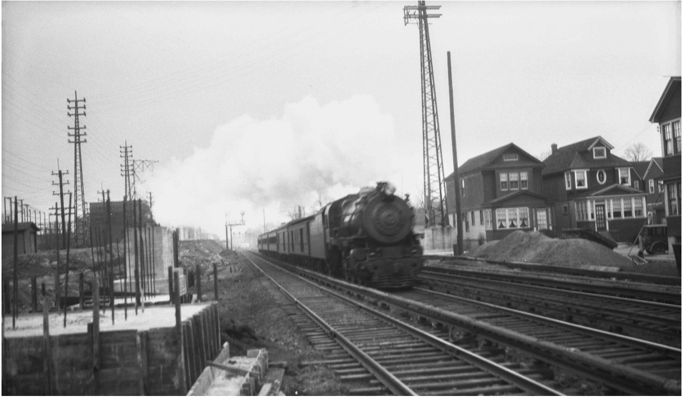
(Above) View west at 175th Street, within the limits of J3 Block Station, just west of Hillside Station. The foundation on the left will support the Montauk Branch viaduct that will cross over the Main Line. (Below) Also looking west, from the pedestrian overpass at Hillside Station, with 177th Street in the foreground. The track on the left is the Montauk Branch turning south to head towards St. Albans, with more of the footings for the future viaduct. This track will split into two tracks just to the east of J3 Block Station, which is just out of view at the bottom left of this picture. The second track from the left is the lead into Holban Yard, the hub of freight operations to the east of Jamaica. The negative of this picture was either poorly exposed or developed, and it needed some work in Photoshop to bring out the image.
