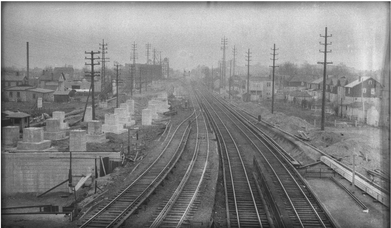
(Above) View west at 175th Street, within the limits of J3 Block Station, just west of Hillside Station. The foundation on the left will support the Montauk Branch viaduct that will cross over the Main Line. (Below) Also looking west, from the pedestrian overpass at Hillside Station, with 177th Street in the foreground. The track on the left is the Montauk Branch turning south to head towards St. Albans, with more of the footings for the future viaduct. This track will split into two tracks just to the east of J3 Block Station, which is just out of view at the bottom left of this picture. The second track from the left is the lead into Holban Yard, the hub of freight operations to the east of Jamaica. The negative of this picture was either poorly exposed or developed, and it needed some work in Photoshop to bring out the image.
