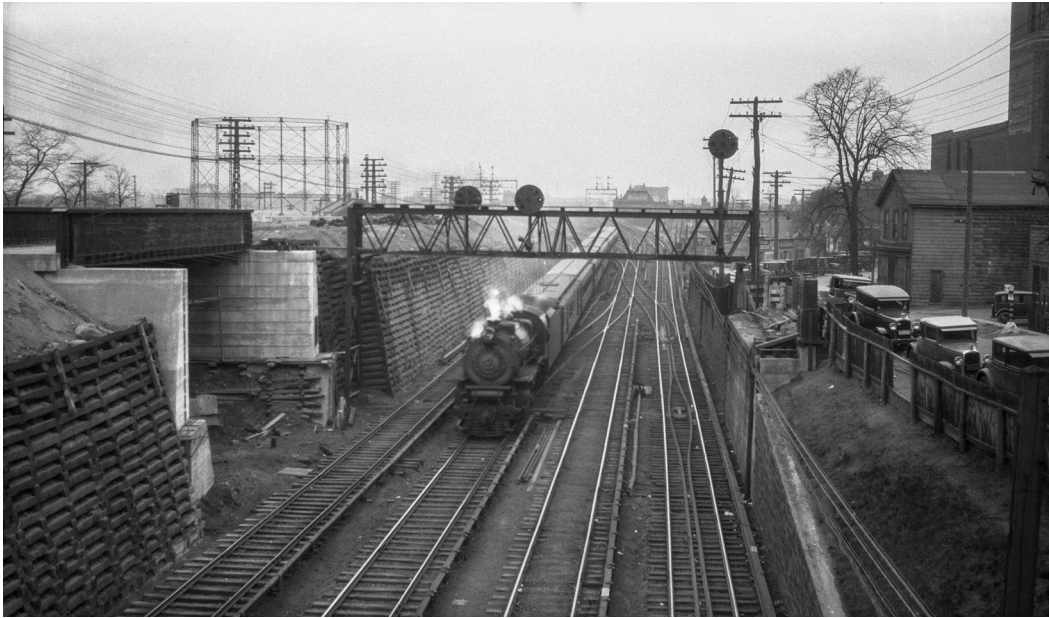
In the view above, Class G5s No. 27 (PRR-Juniata, 1/1925, s/n 3976) is leading an eastbound train on Track 3 at 159th Street. The track immediately to the right of the train stub-ended at the high-level platform of Union Hall Street Station. The temporary J1 Block Station is barely visible on the right, through the signal bridge. Below, class D16sb No. 223 (PRR-Juniata, 2/1906, s/n 1444) leads a westbound train through the switches of J2 Block station, at 170th Street. The overpass in the distance is at Hillside Station.
