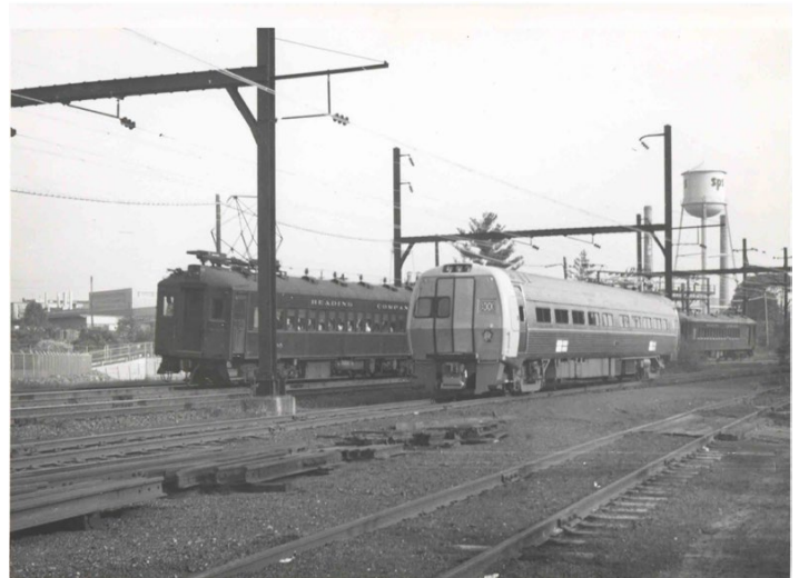
Metroliner production coach car #800 along the Reading Railroad's New York Branch shortly after delivery by Budd in 1967. This was the first car equipped with Westinghouse propulsion delivered. The Metroliner cars would later cause problems with the Pennsylvania Railroad MP-54 fleet (later Penn Central) by blowing out the old cars' windows when passing an oncoming train at high speed. ERA Collection.
