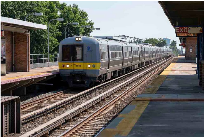
M3 No. 9895 (Budd-GE, 9/1986) leads Train No. 1927 from Ronkonkoma to Penn Station through Floral Park Station at high speed on July 23. The platform on the right has several pieces of plywood covering damaged portions of concrete. Jeff Erlitz photo
