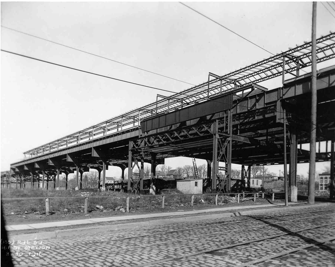
Mr. Manchester is standing on the south side of 161st Street and west of River Avenue. This is looking northeast at the mezzanine and what will be the stairways down to the street. Note the tracks of the 163rd Street Crosstown trolley in what is now only the eastbound lanes of 161st Street. Like at Mosholu Parkway Station near the end of this line, this mezzanine and street stairs will be clad in concrete. Charles Manchester/PSC photo
