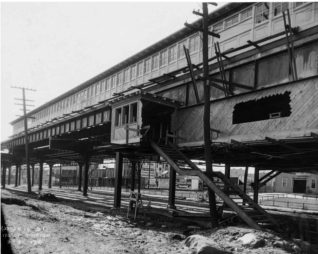
Looking southwest from the south curb of East 170th Street, off Jerome Avenue. The windows along the outer edges of this platform have been installed and the woodwork of the mezzanine is well under way. Note that the hole cut out for the mezzanine window has only been partially trimmed for the eventual installation of the windows. Charles Manchester/PSC photo
