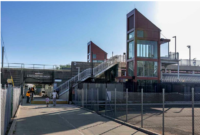
View northeast of the new elevators, at the west ends of the platforms. Glen Sager/MTA photo
