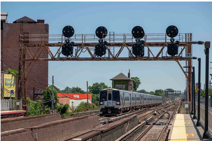
Also on July 23, M9 No. 9045 (Kawasaki Rail Car, 8/2020) is on the point of Train No. 1533 (Huntington-Penn Station) and is about to pass under Signal Bridge No. 1 at the east end of Queens Village Station. This signal bridge, the only one remaining in Queens Interlocking from the original 1924 grade separation project here, is being kept. The new Reduced Aspect Signals were mounted in back of the lower "arms" of the position light signals. Jeff Erlitz photo
