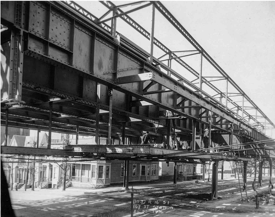
Looking north from just east of the southeast corner of River Avenue and 167th Street, the steelwork for the mezzanine appears to be nearly complete. The wooden structures on the far corner have long since been replaced with single-story commercial brick buildings. Charles Manchester/PSC photo
