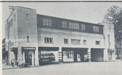
IRT Station - Woodlawn - Jerome Ave. Line
