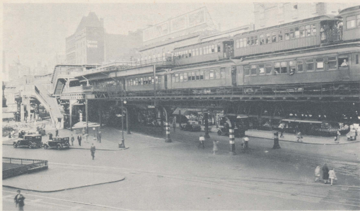
A Ninth Avenue uptown express rises above a downtown Sixth Avenue local at 66th Street. This appearance was the same at most express stations on the 2nd, 3rd and 9th Avenue lines. (N.Y.C.T.A. Photo)
