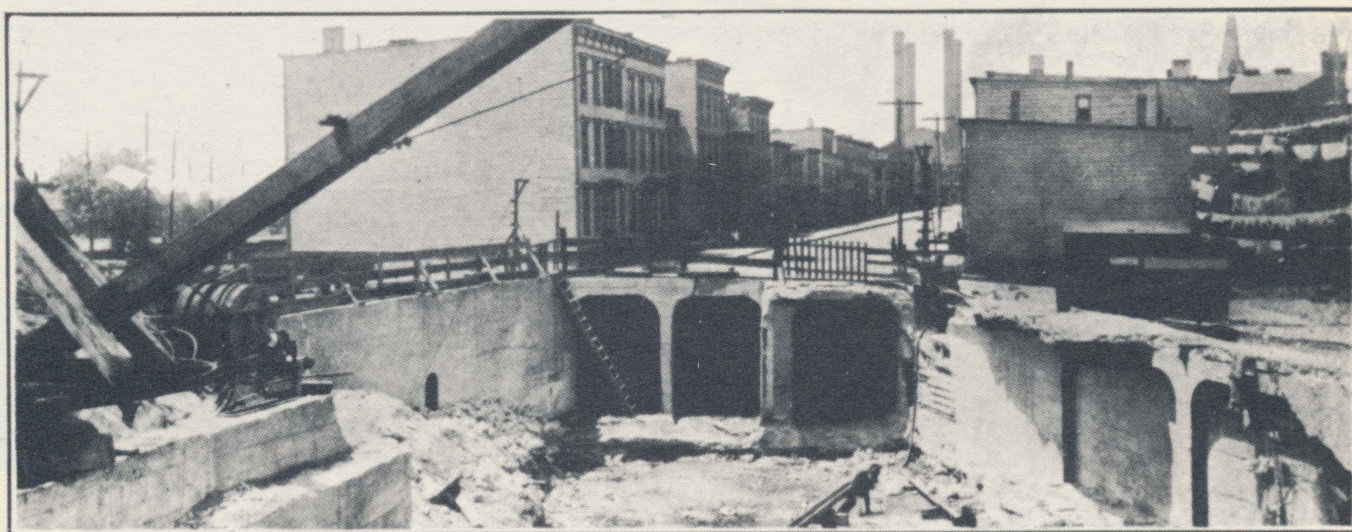
RECONSTRUCTION WORK AT MOUTH OF STEINWAY TUNNEL IN LONG ISLAND CITY. PHOTO TAKEN JUNE 6, 1914.
