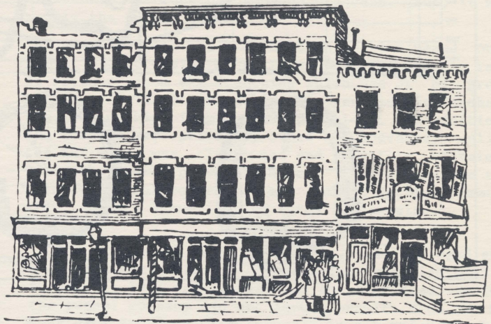
FRONT OF THE ROW OF SHATTERED BUILDINGS.
