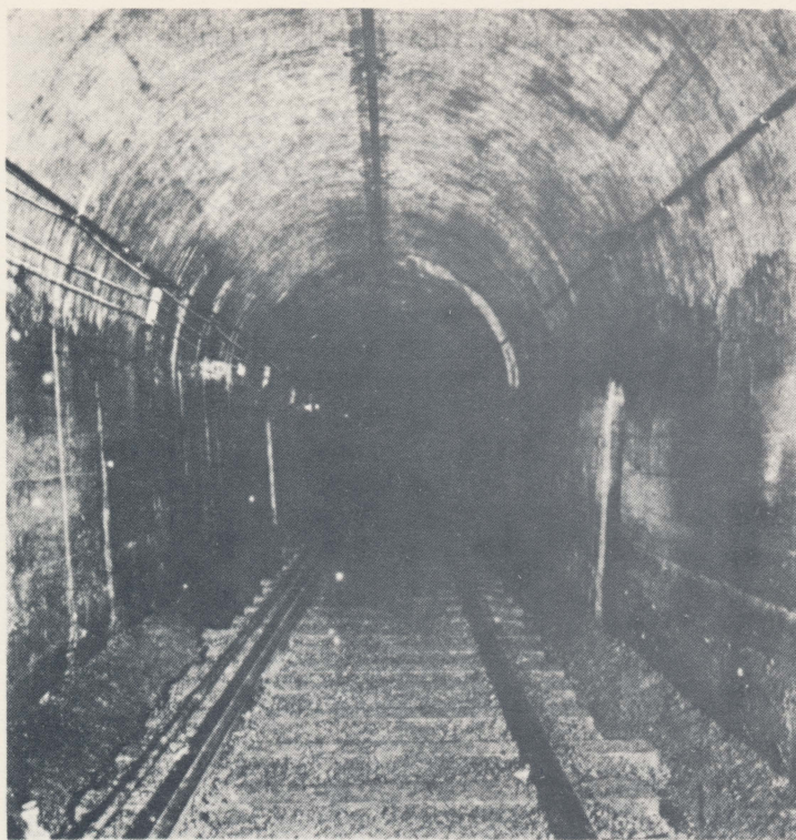
INTERIOR VIEW OF CONCRETE SECTION OF THE FORTY- SECOND STREET TUNNEL, SHOWING OVERHEAD CON- TACTOR, ROADBED, ETC.
