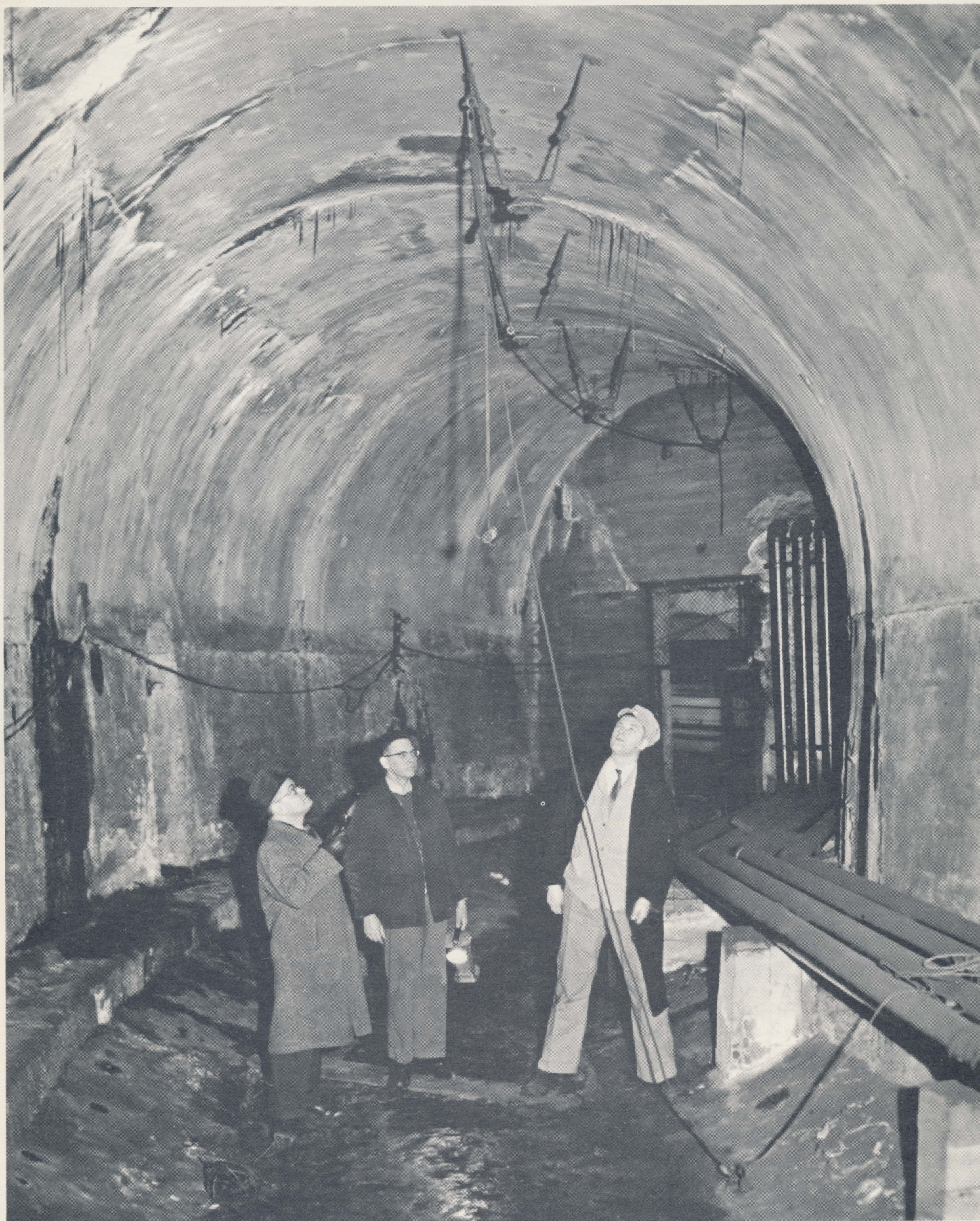
In this photo, taken for ELECTRIC RAILROADS , author David Rogoff, Bill Chamberlain of the TA, and editor George Horn inspect old third rail bracket hanging from ceiling of former trolley car loop just west of Grand Central station. Blur in background doorway is Queens-bound train. Pipes on right are for drainage purposes and are of recent origin. (Roland Harvey photo)
