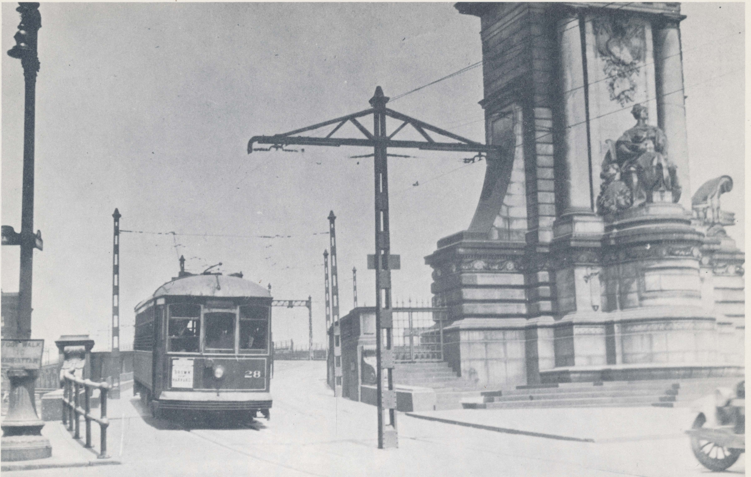
The monumental entrance at the Brooklyn Plaza of the Manhattan Bridge caused an 'S' curve in the 3¢ Line trackage, site of the 1923 accident. The car shown was constructed by Southern Car Company, the sculpture by Daniel Chester French, of 'Brooklyn'
