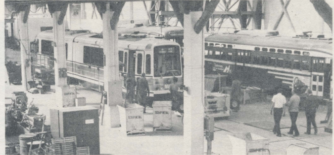
LRV No. 1220 and PCC's No. 1027 and 1020 are seen here at Muni's new Metro Center, built on the site of the former Elkton Shops. --San Francisco PUC
