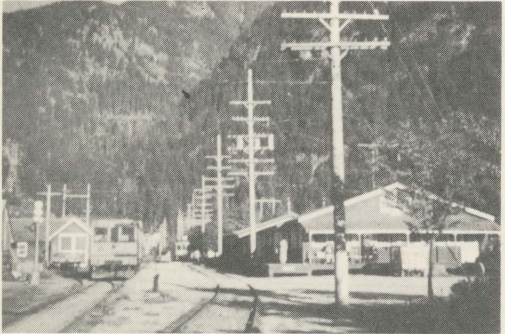
8. New Halem HQ, 89 on main, ex. Oregon Electric Interurban on siding beyond platform.
